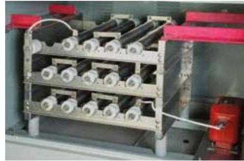
An example of a neutral ground resistor (courtesy I-Gard)
