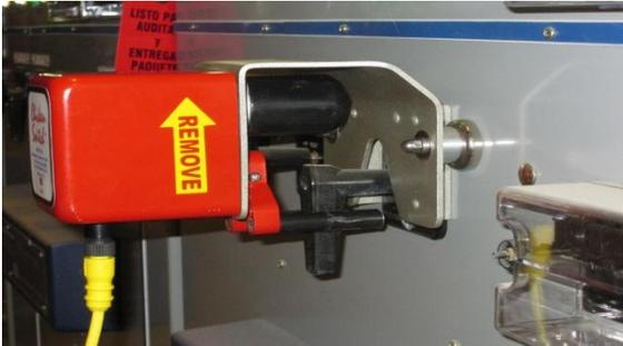
This remote switching device utilizes an actuator to operate the control handle, allowing operating personnel to stand outside the boundary of the arc flash hazard. Without the remote switching device, the person would be standing in close proximity to the switchgear.
