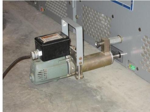
This motor operated device allows the removal or insertion of a draw-out circuit breaker. The person can stand outside the boundary of the arc flash hazard. Without the remote operator, the person would be kneeling in front of the switchgear using a manual wrench.
