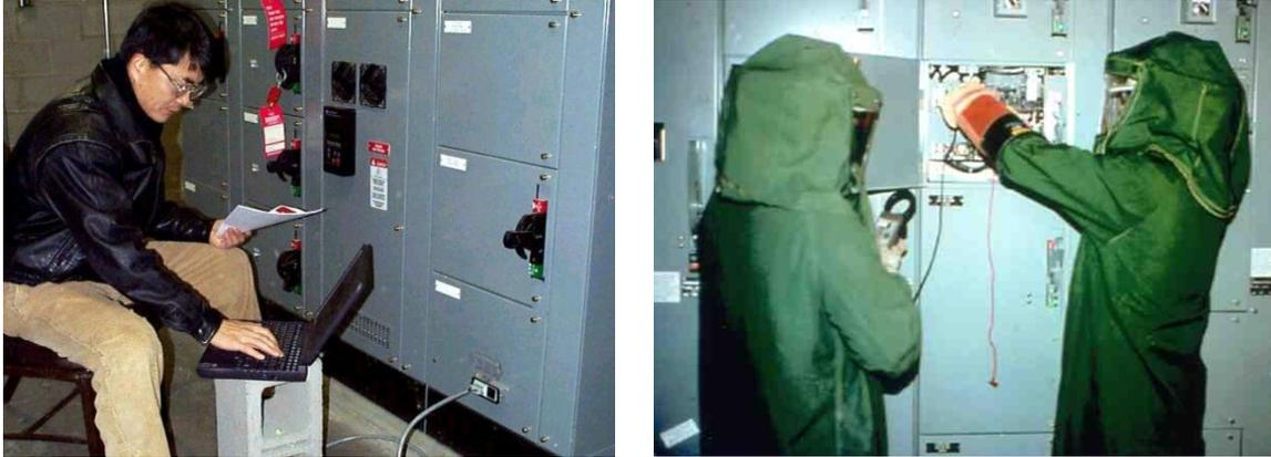
**Figure 13. The motor control center on the left has “smart” technology, including sensors and data highway that enables the technician to perform troubleshooting and adjust protective device settings without opening enclosure doors, avoiding exposure to unguarded energized components. The motor control center on the right does not have the “smart” technology. Troubleshooting must be done using chock and arc flash PPE to protect the workers from hazards from unguarded energized components.**
