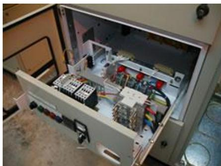
**Figure 10. A fully withdrawable motor control center design. The motor starter is shown in the withdrawn (disconnected) position.**
