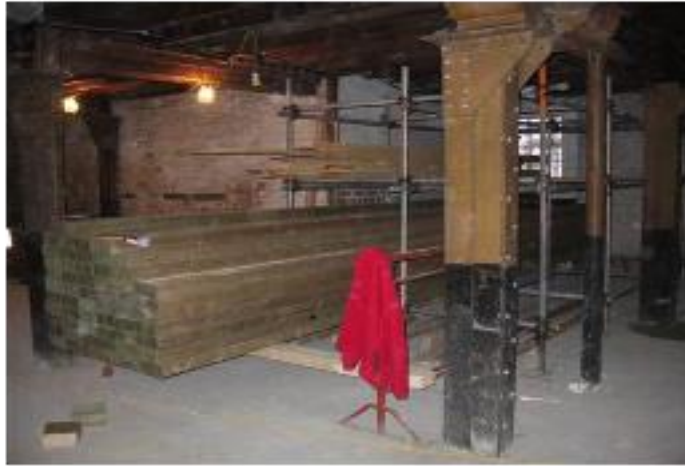
A designated timber storage area
