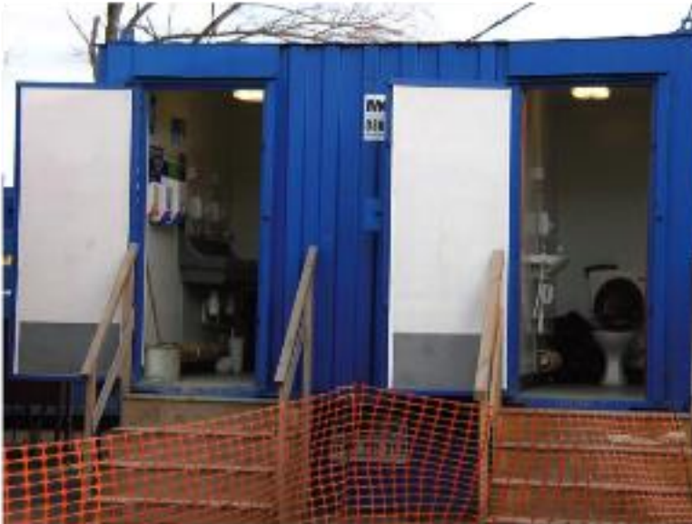
A self-contained water-flushing toilet block with built-in tank
